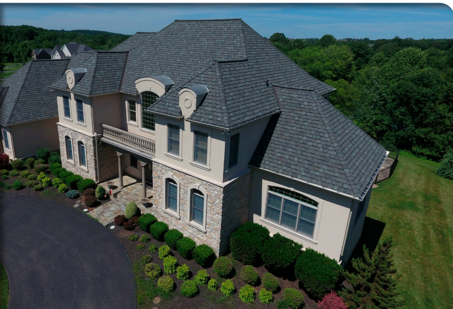
Drone shot of a roof installation completed in early 2016.
