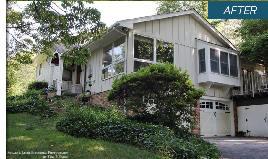
Before and After photos of a James Hardie installation completed by American Home Contractors.
